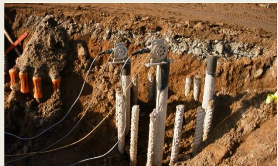
SONIC LOGGING (PILE INTEGRITY)
