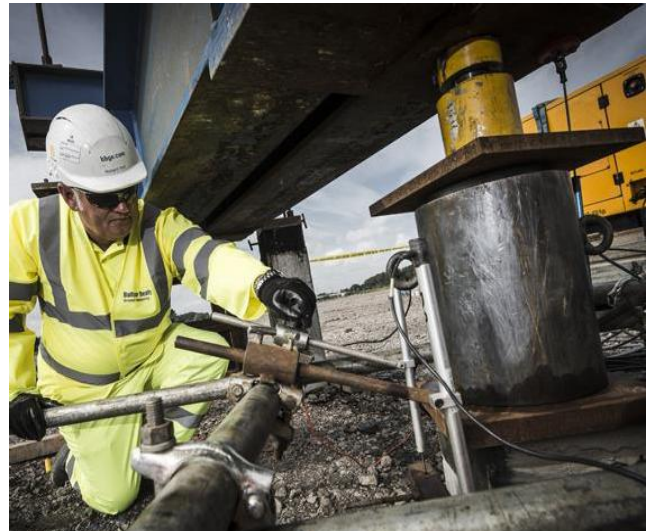
STATIC LOAD PILE TESTING
