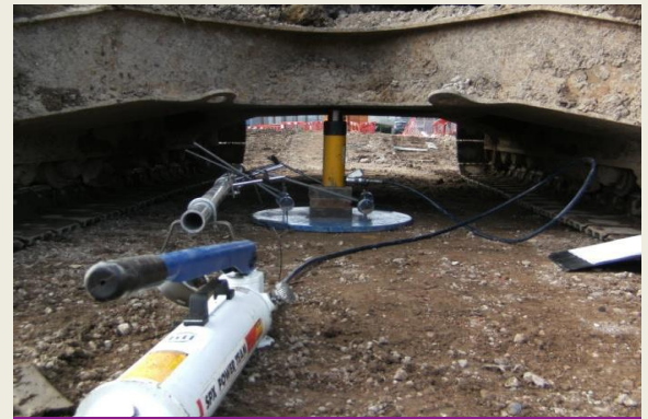
PLATE LOAD PILE TESTING
