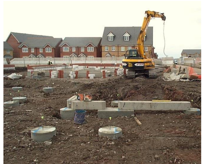
PILE CAPS IN PLACE & BEAMS BEING LAID
