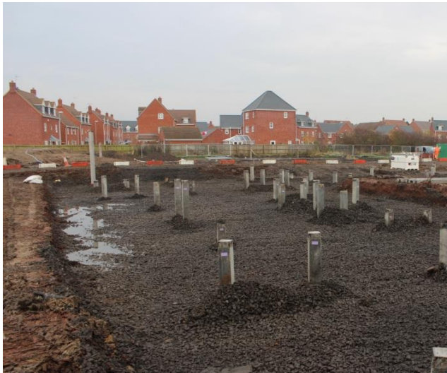
PRECAST PILES DRIVEN TO DESIGN LENGTH
