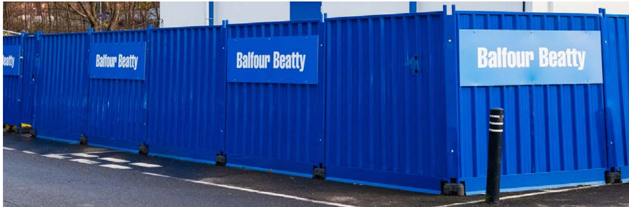
Standard approach on metal hoardings
