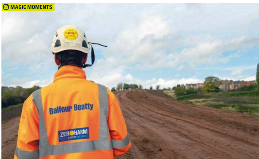
UK: Gedling Access Road, Nottinghamshire County Council. Photo credit: Paul Stephenson
