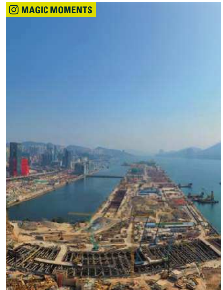
Hong Kong: Central Kowloon Route - Kai Tak West, Highways Department, HKSAR Government. Photo credit: Lunggy Fung
