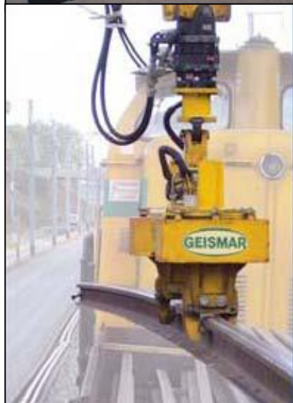
Typical Rail lifting beams
