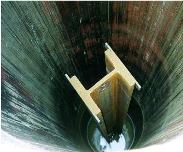
PLUNGE COLUMN EMBEDDED IN CONCRETE AT DEPTH
