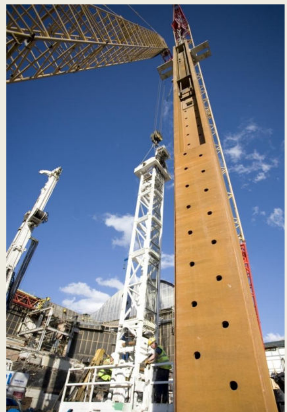
INSTALLATION OF PLUNGE COLUMNS
