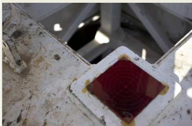
LASER SYSTEM ENSURES HIGH LEVEL OF VERTICAL ACCURACY
