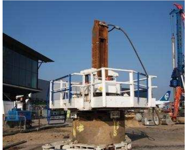
COLUMN AND FRAME ARRANGEMENT – BORED PILING
