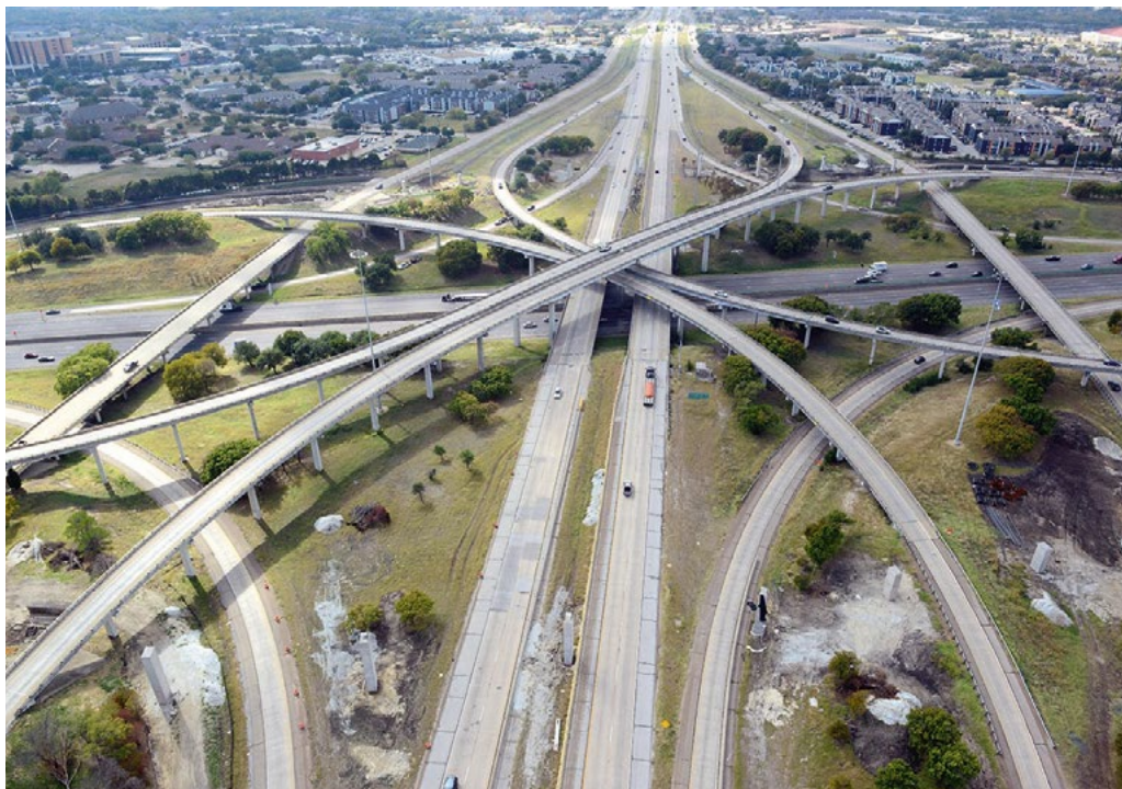
LEFT: The Southern Gateway reconstruction and improvement project for the Texas Department of Transportation, US.
