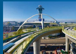
US: Automated People Mover, Los Angeles International Airport.
