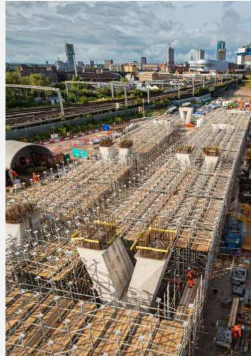
Deck span for Curzon St viaduct
