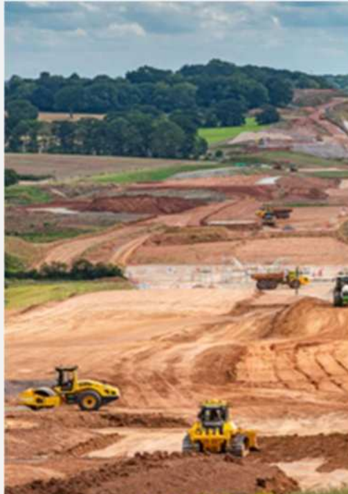
Cubbington cutting earthworks
