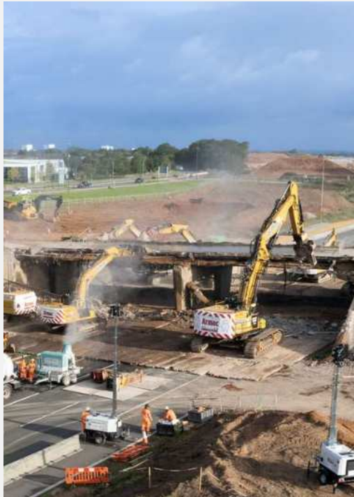
M42 bridge demolition
