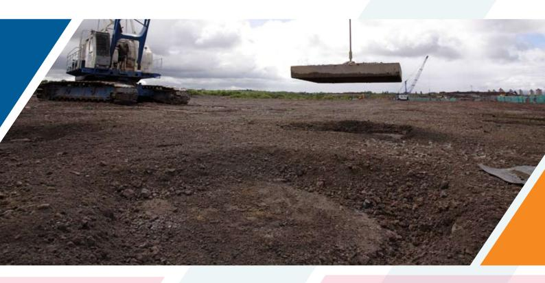
Dynamic Compaction (DC) is the use of high energy tamping to induce settlement in a wide variety of ground conditions from loose granular materials to mixed made ground, including domestic landfills.
