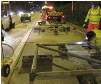
Stage 2 - Resin anchored sockets are installed and holes are drilled for grouting
