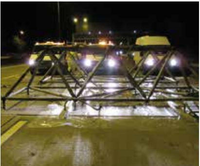
Stage 3 - The carriageway is lifted and grouting commences
