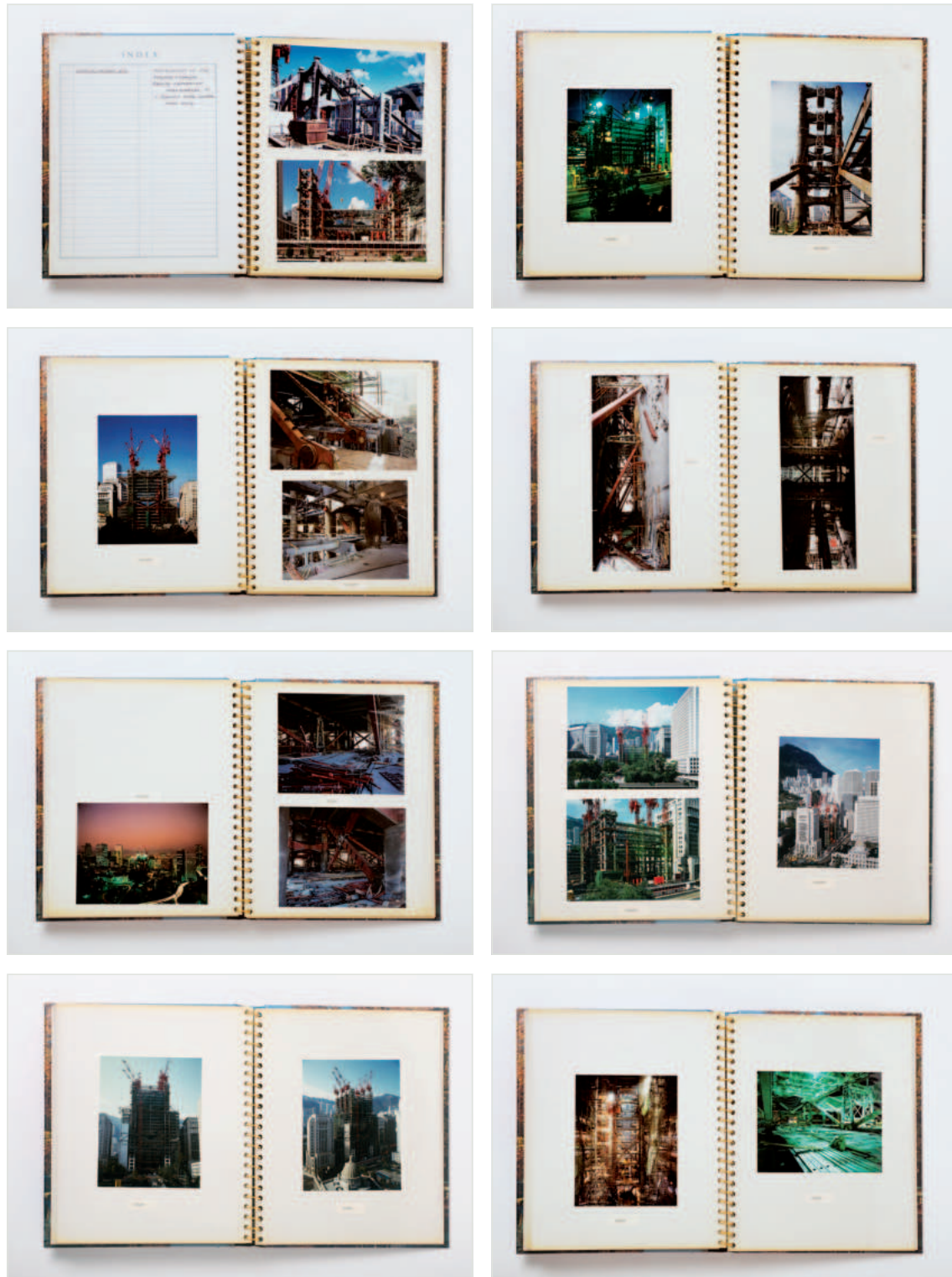
Above: Work in progress photograph album, 1983-1984. Right: The project approaches completion.
