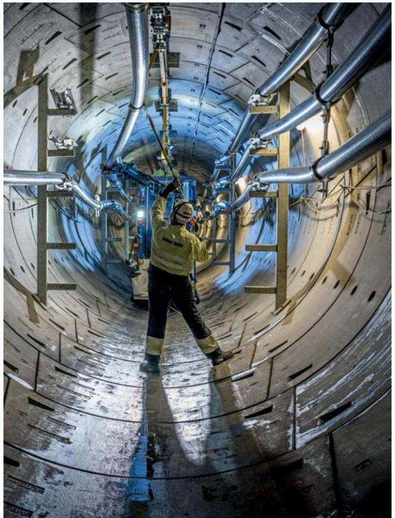
We're installing high-voltage electricity cables in deep underground tunnels, protecting London's future demand for energy.
