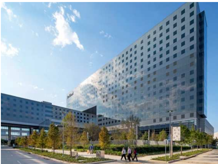
We recently completed the largest healthcare project in the US: the New Parkland Hospital in Dallas is a 1.9 million sq ft 862-bed hospital.
