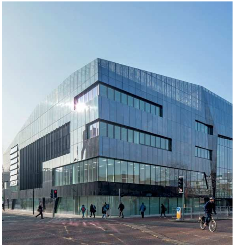
We delivered mechanical, electrical and process services for the leading edge facility that will carry out detailed research into Graphene.
