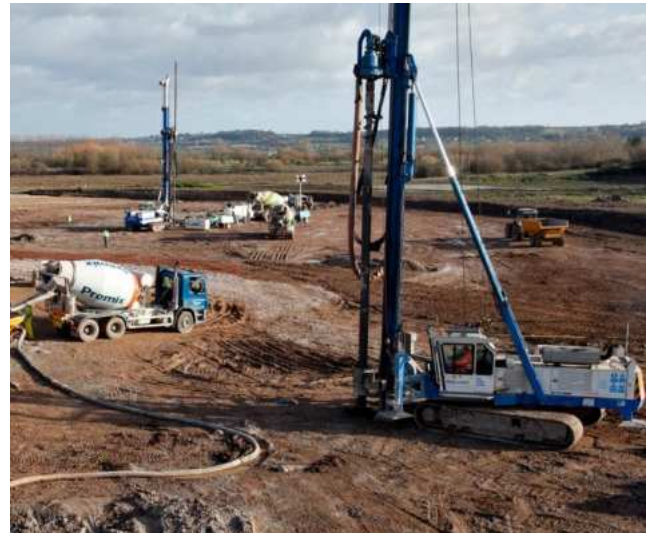
MULTIPLE RIGS WORKING ON SITE
