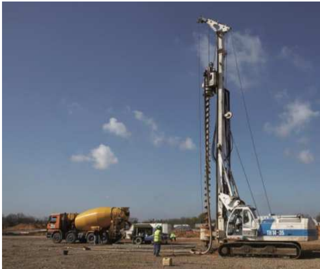
INSTALLATION OF PENCOL COLUMNS
