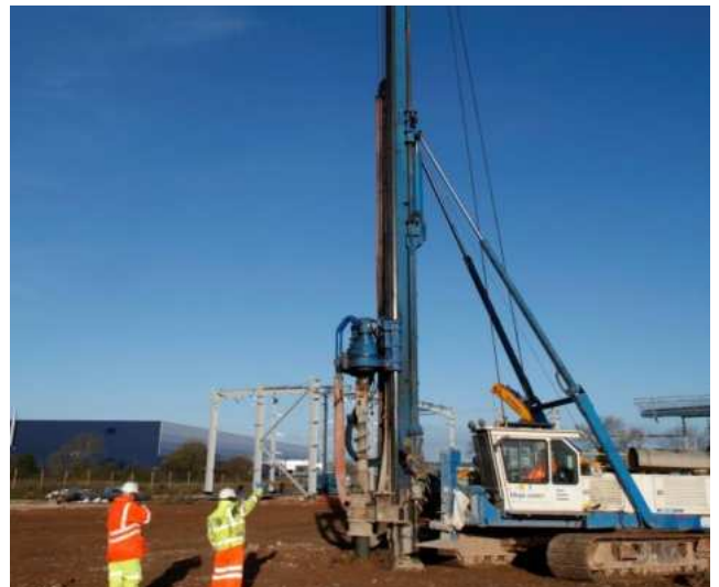
PENCOL INSTALLATION - AUGER DISPLACEMENT TECHNIQUE
