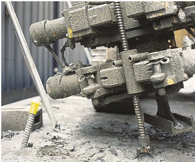
SELF-DRILL MICROPILE WITH CLAY BIT
