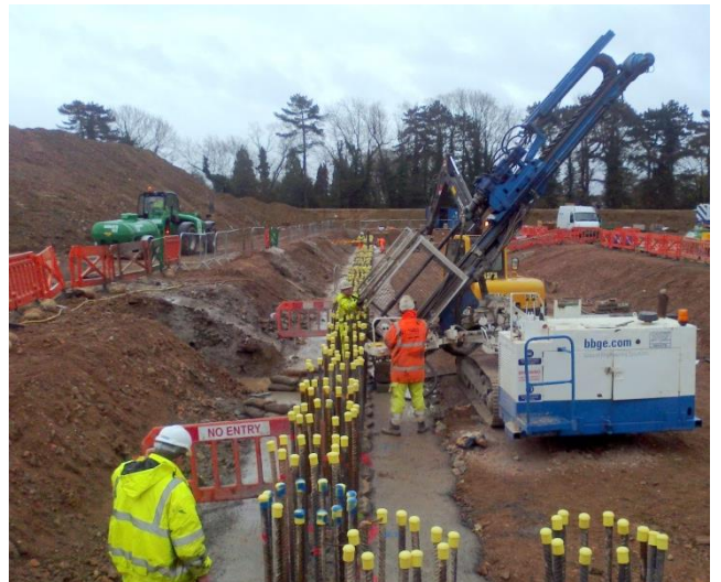
INSTALLING SELF DRILL ANCHORAGES
