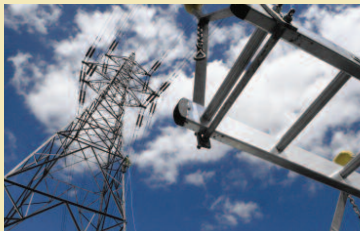
Eastern Electricity Alliance
