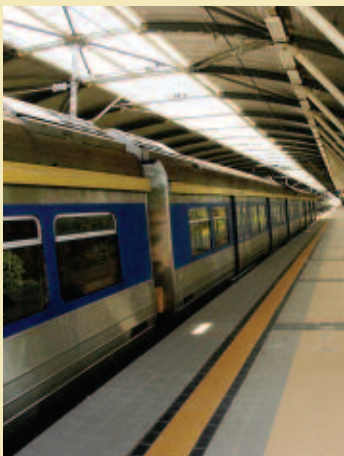
Rawang-Ipoh Electrification, Malaysia
