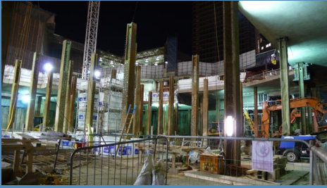
Excavation showing ring beam
