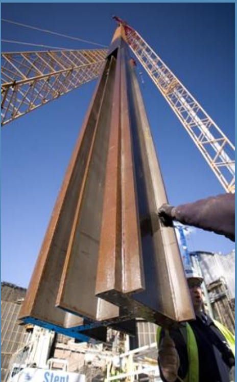
Plunge Column with fins To increase surface area
