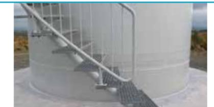
Repaired turbine base following embedded CAN stabilisation, concrete repair and resealing
