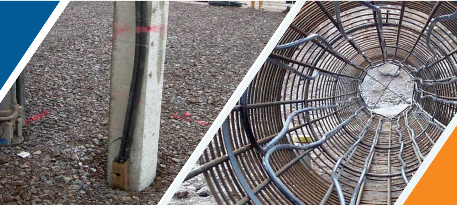
Providing Geothermal Piles for use in ground storage systems is one way that Balfour Beatty Ground Engineering (BBGE) can help with the provision of renewable energy and reduce carbon emissions.
