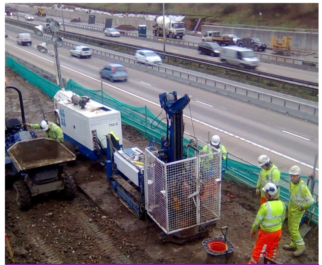
RESTRICTED SPACE CAPABILITY WITH SAFETY CAGE IN PLACE
