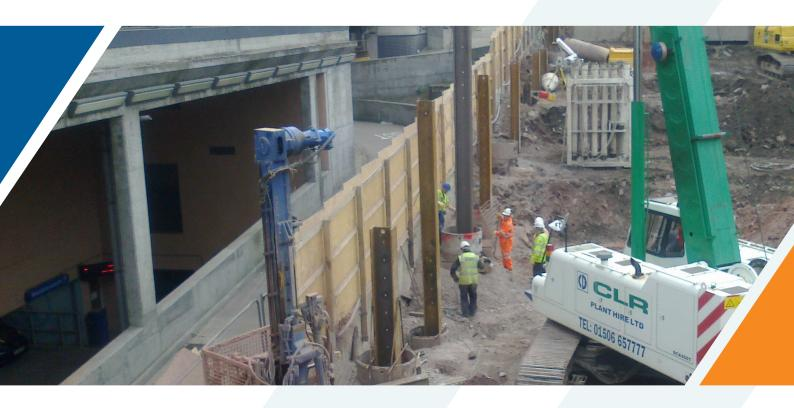
King post walls are a cost effective earth retention system, either as a permanent or temporary solution, which can be constructed using concrete panels, timber sleepers or beams, or steel panels.
