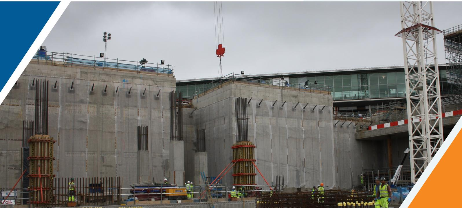
Diaphragm walls are underground structural elements commonly used as retention systems and permanent foundation walls. They can also be used as groundwater barriers.
