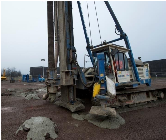
SOME HEAVE DURING INSTALLATION PROCESS
