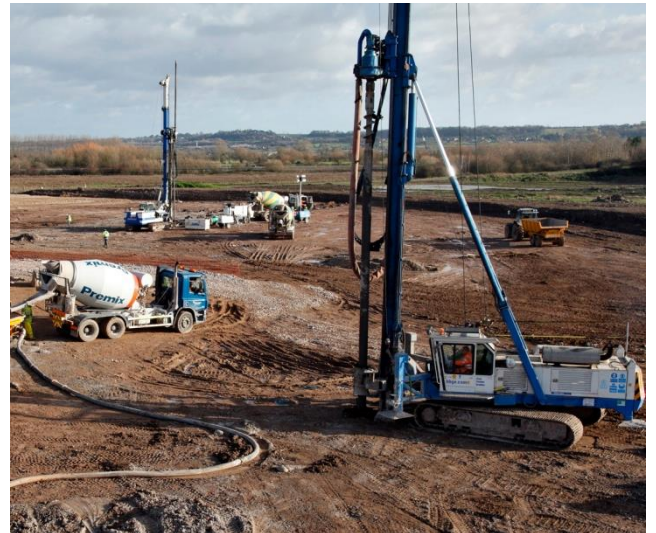
MULTIPLE RIGS WORKING ON SITE
