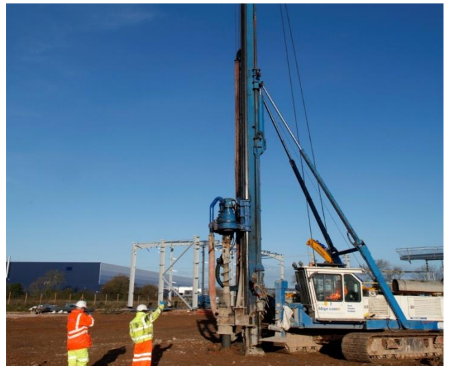
PENCOL INSTALLATION - AUGER DISPLACEMENT TECHNIQUE
