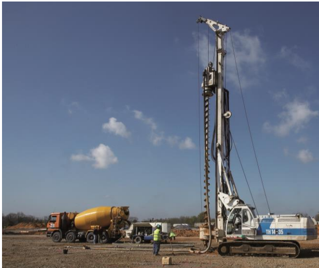
INSTALLATION OF PENCOL COLUMNS
