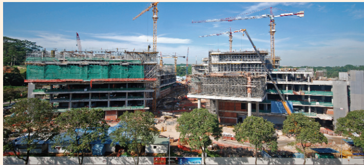
Construction is underway at The Institute of Technical Education in Singapore
