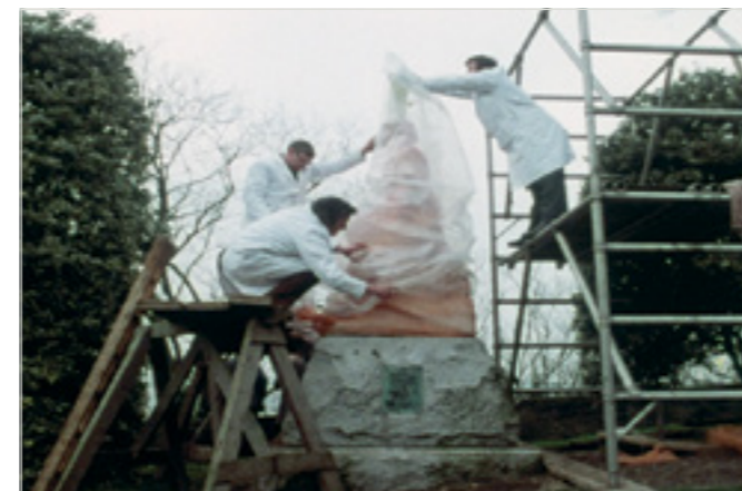
Top: Colquhoun-Moran cavity lining in load bearing test. Above: Statue of Lady Jerningham being given the Balvac treatment – from Tomorrow's World, 1975. Left: A sprayed concrete gun, 1955.
