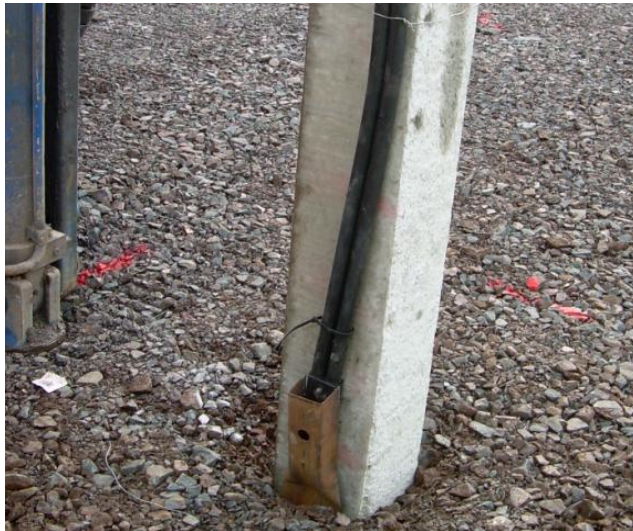
GEOHERMAL SYSTEM INSTALLED ON PRECAST PILE
