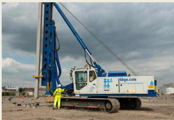
PRECAST PILE INSTALLATION
