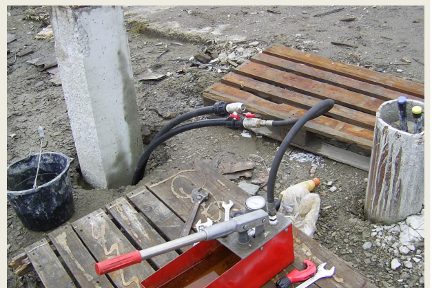
GEOHERMAL LOOP PRESSURE TESTING
