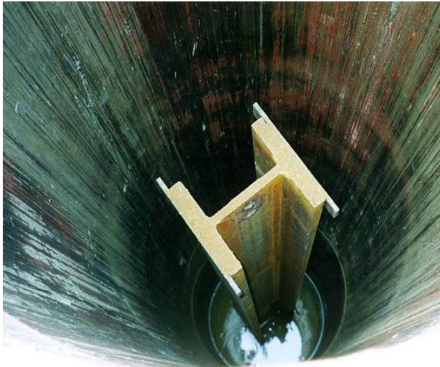
PLUNGE COLUMN EMBEDDED IN CONCRETE AT DEPTH
