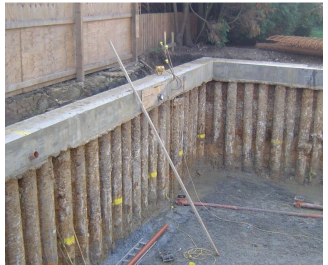
CONTIGUOUS MINIPILED RETAINING WALL
