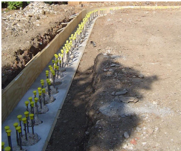
ROW OF INSTALLED AUGERED MINIPILES
