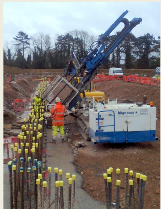
INSTALLING ANCHOR PILES
