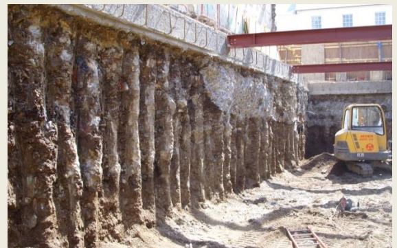
CONTIGUOUS MINIPILED RETAINING WALL
