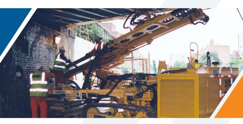
Ground Anchorages are used for a variety of applications and take a number of forms with uses for both temporary and permanent works. Simplistically they are anchorages into the ground which can be either passive or active in type.
