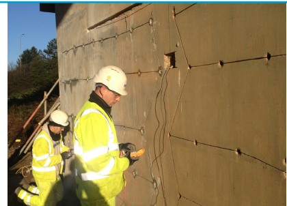
Testing CP during installation on the A47 Paston Interchange
