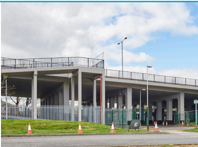
Anlaby road flyover refurbishment, Hull
