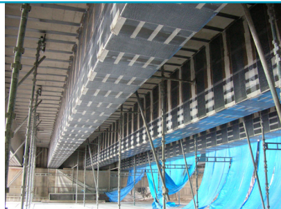
Carbon fibre bridge strengthening, Corkerhill Road Bridge
