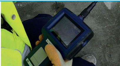
Endoscope inspection of anchor ring
