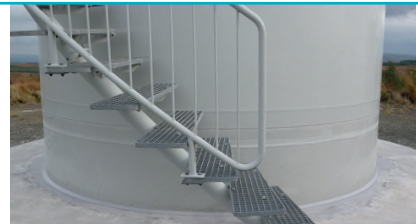
Repaired turbine base following embedded CAN stabilisation, concrete repair and resealing
