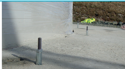
Injection packers fixed prior to embedded CAN stabilisation works
