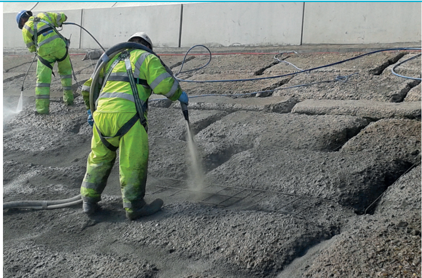
Spray concrete repairs to revetments at Grimsby
