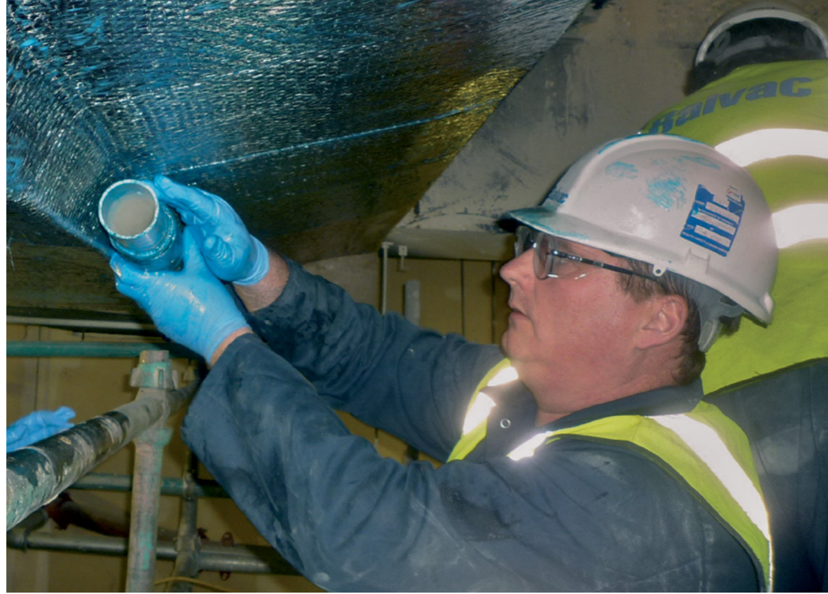
Right: Installation of carbon fibre wrap at Gatwick Airport
