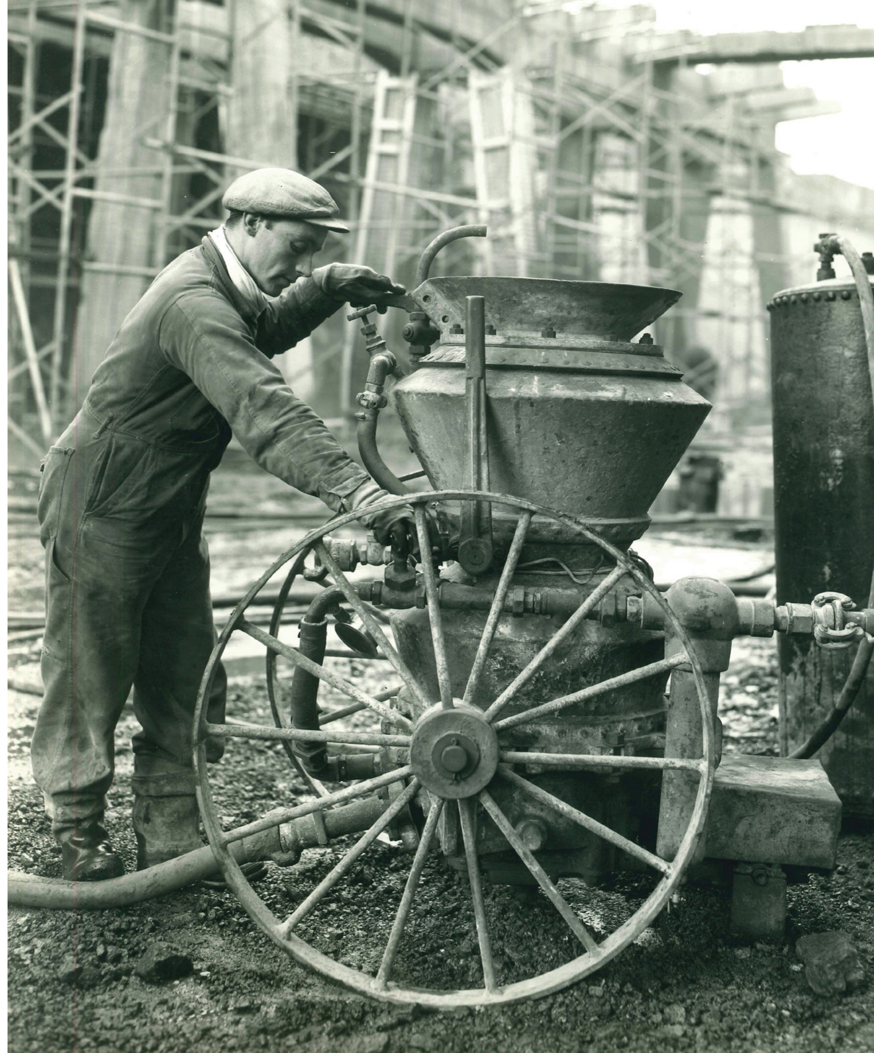
Below: Sprayed concrete roof, Barclays, Warrington
