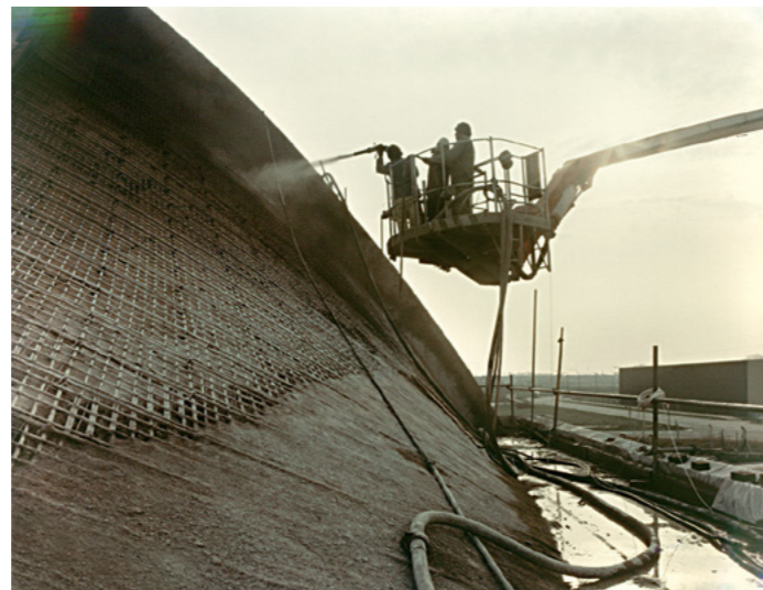
Opposite: Sprayed Concrete Gun, March 1955
