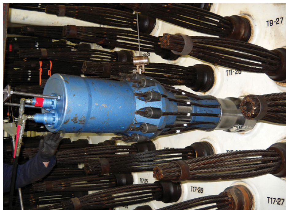
Right: Tendon monitoring at Oldbury Power Station Opposite: Repairing the Castlefield Viaduct in Manchester
