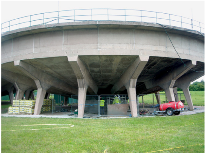
Right: Concrete repairs at the Chester sewage treatment works Opposite: 'Top of the Cow' – Post tension installation as part of tank construction
